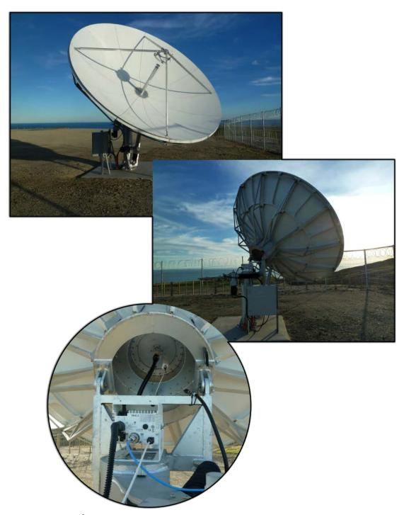
Figure 3.2 IBUC 2 Field Installation
